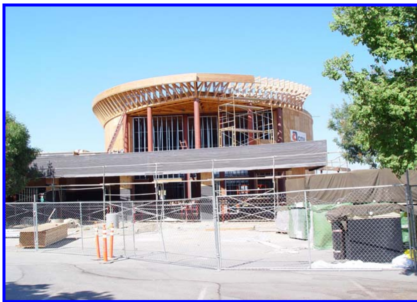
City Hall Council Chambers under construction
