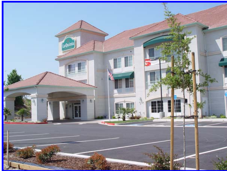
Located at the Jack Tone Interchange
