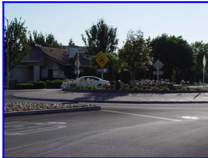
Single lane roundabout on Doak Boulevard
