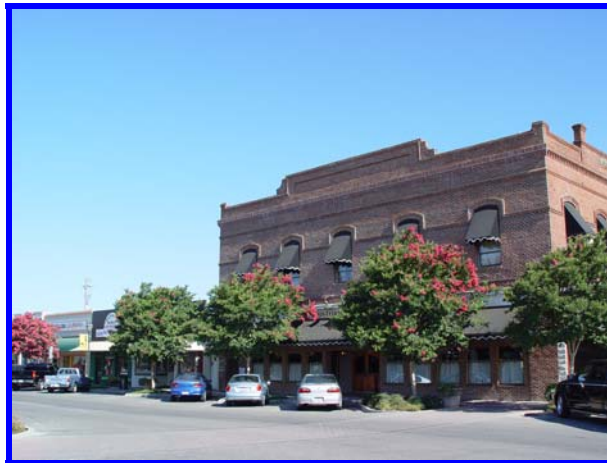
The Old Odd Fellows Building located on E. Main Street
